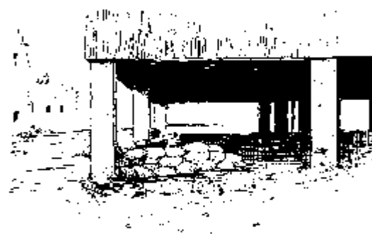
Position with overhead cover
