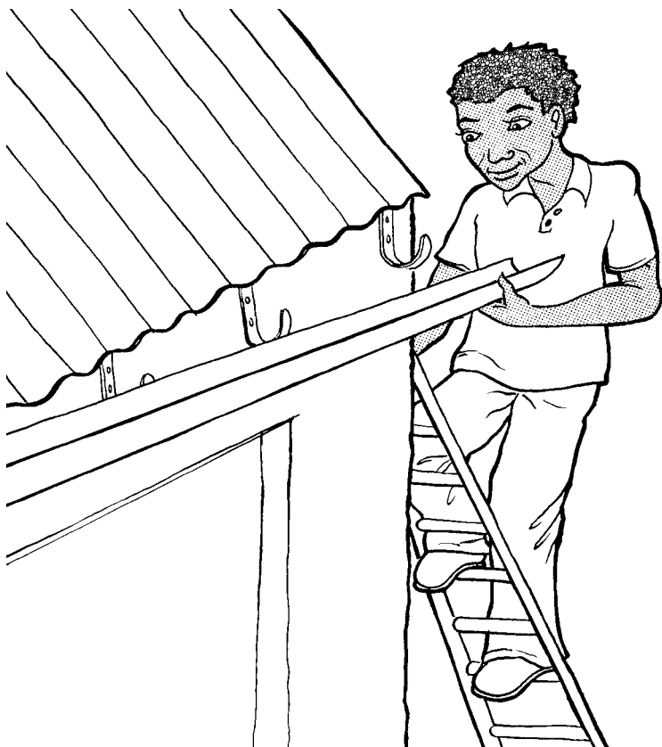
Figure 4: Connecting a gutter system
